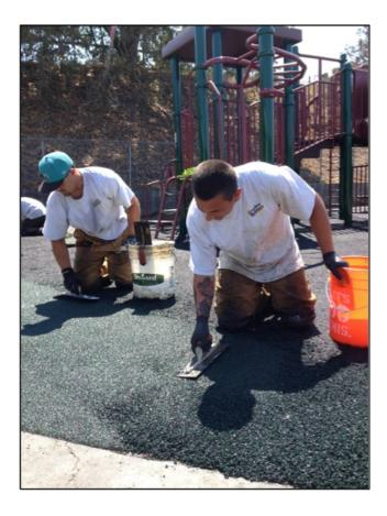
Creative Builders staff lay down a rubber surface which replaces wood chips around the play structure. The rubber pad is
